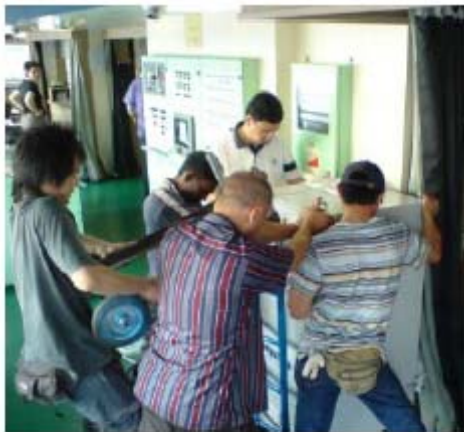
Fig 8. Installation of SIU
