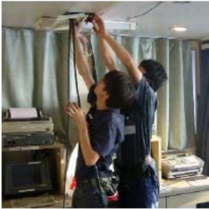
Fig 7. Installing cables for SIU
