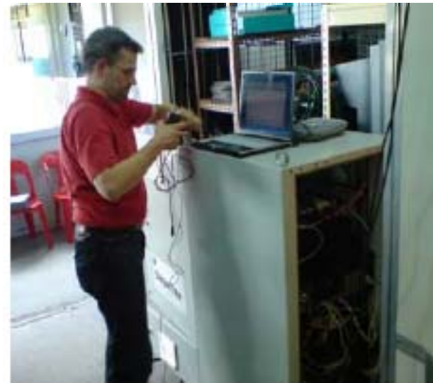
Fig 2. Getting ready to work on the SIU on 5 Mar 07.
